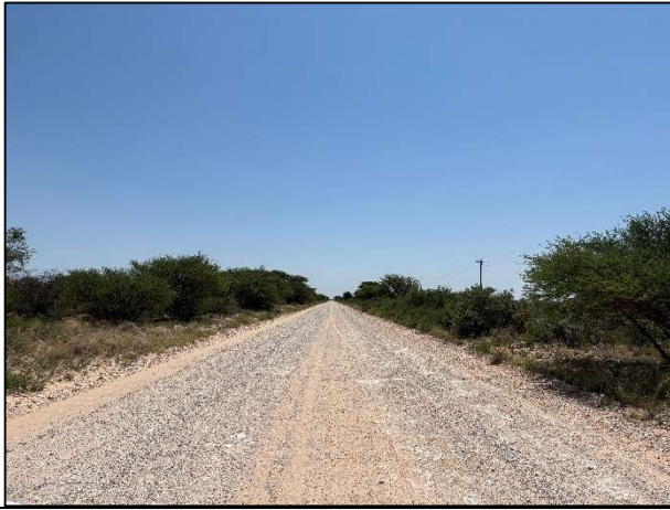
Photo 3: The thoroughly compacted and disturbed road surface typical of the proposed development surface area at photo location 3.
