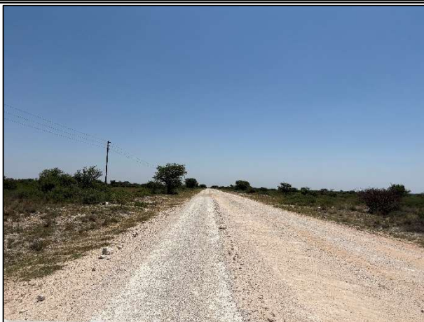
Photo 1: The thoroughly compacted and disturbed road surface typical of the proposed development surface area at photo location 1.
