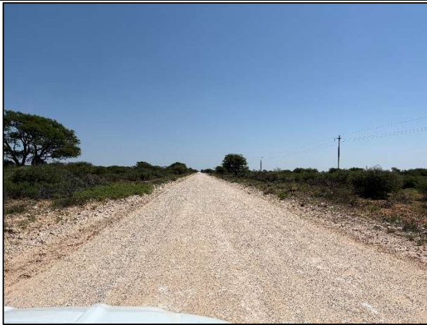
Photo 5: The thoroughly compacted and disturbed road surface typical of the proposed development surface area at photo location 5.
