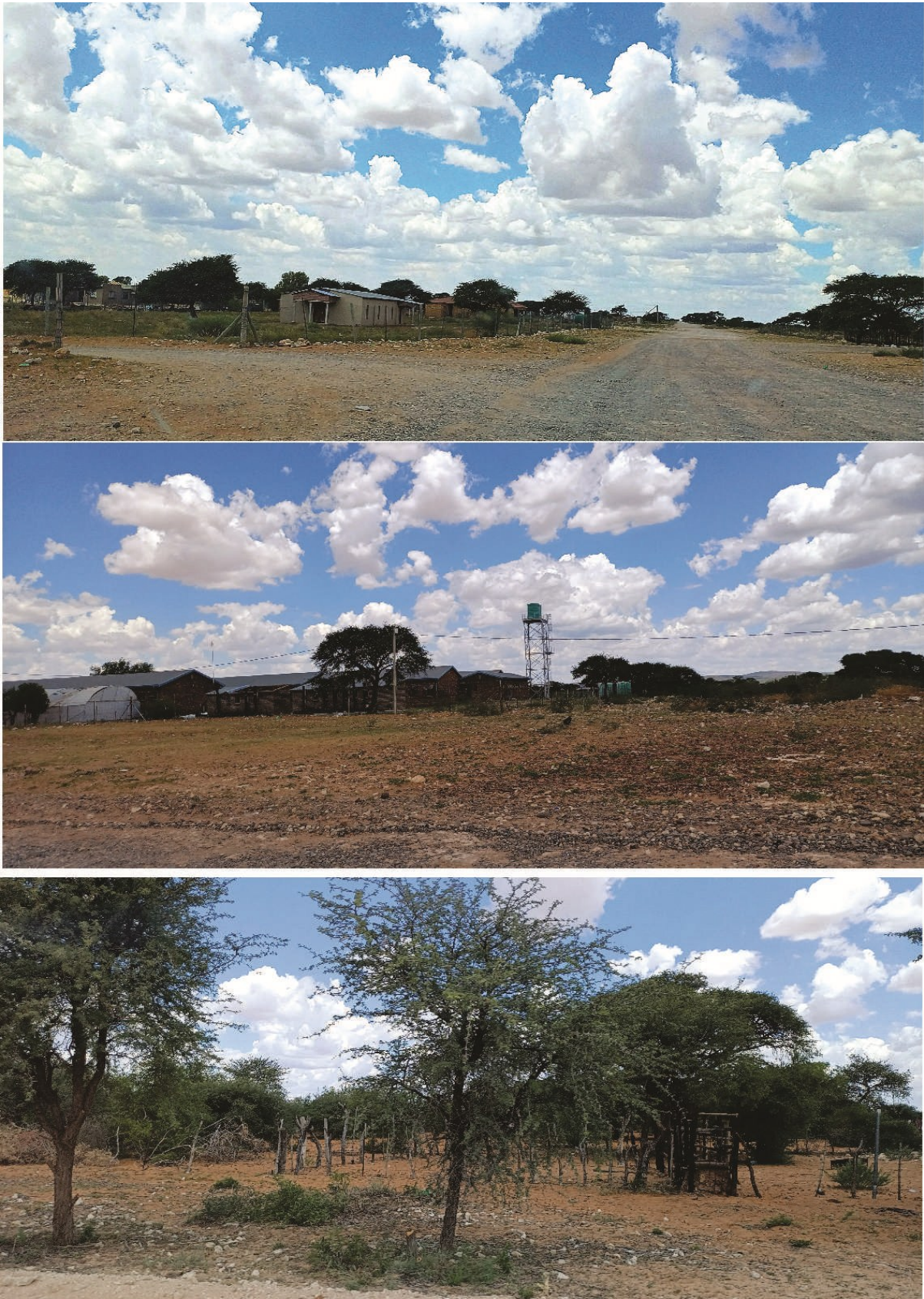
Figure 8. Modern man-made structures situated near or within the vicinity of the road reserves.
