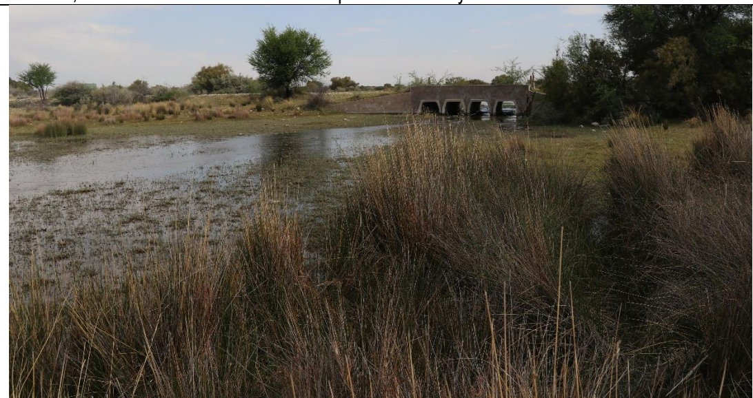
The existing crossing contains several culverts, which are still likely to result in some constriction of flow. Note abundance of flow, even at the end of the dry season, which indicates that the system is likely to be almost perennial.
