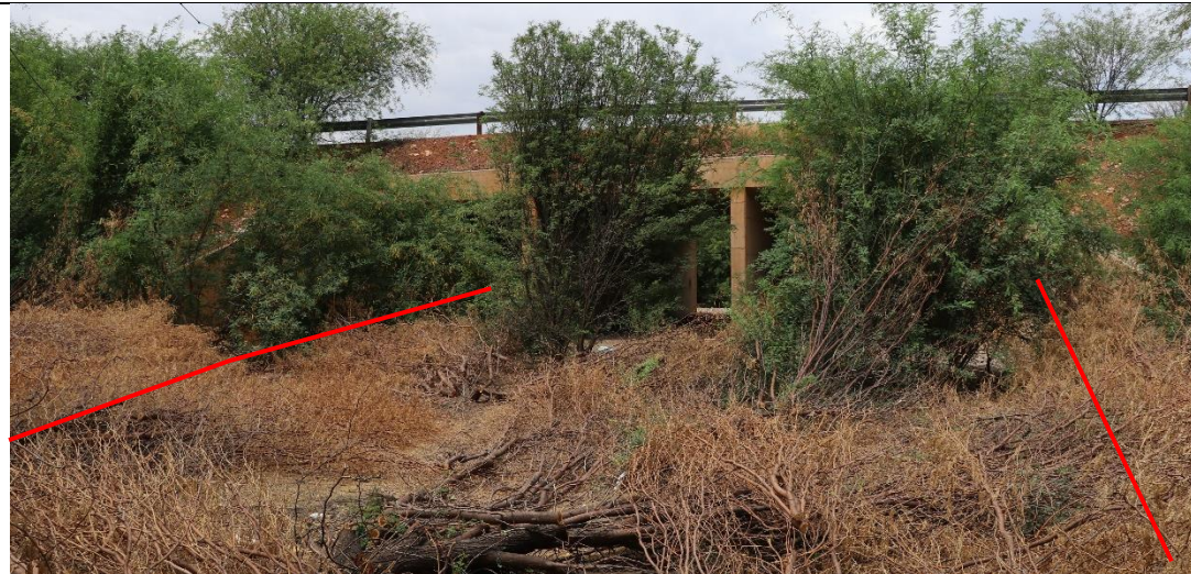
View of the main channel (Red), which is fairly narrow, with an extensive infestation by invasive Prosopis glandulosa also evident. The bridge structure is also clear.
