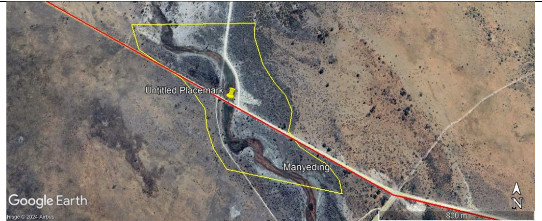
View of the Manyeding River (Yellow), draining from the plains to the south and being crossed by the existing road (Red). Note a prominent channel and fairly extensive floodplain.
