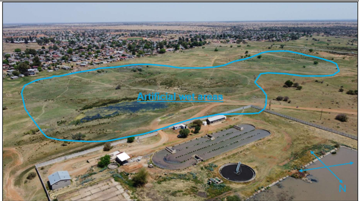
(Drone photo taken at the existing WWTW)
