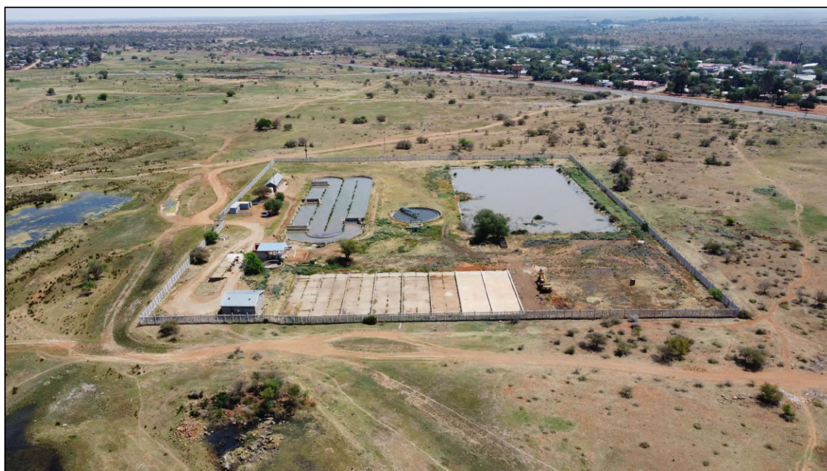
Figure 23: Aerial view of the existing WWTW.
