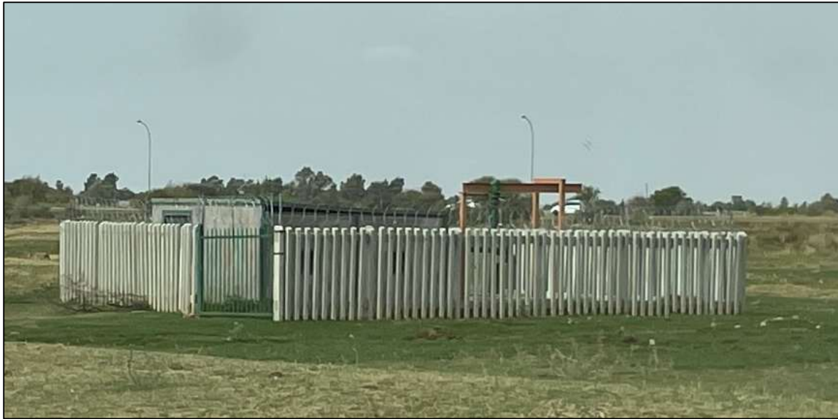
Figure 4: Example of a fenced lift station:
