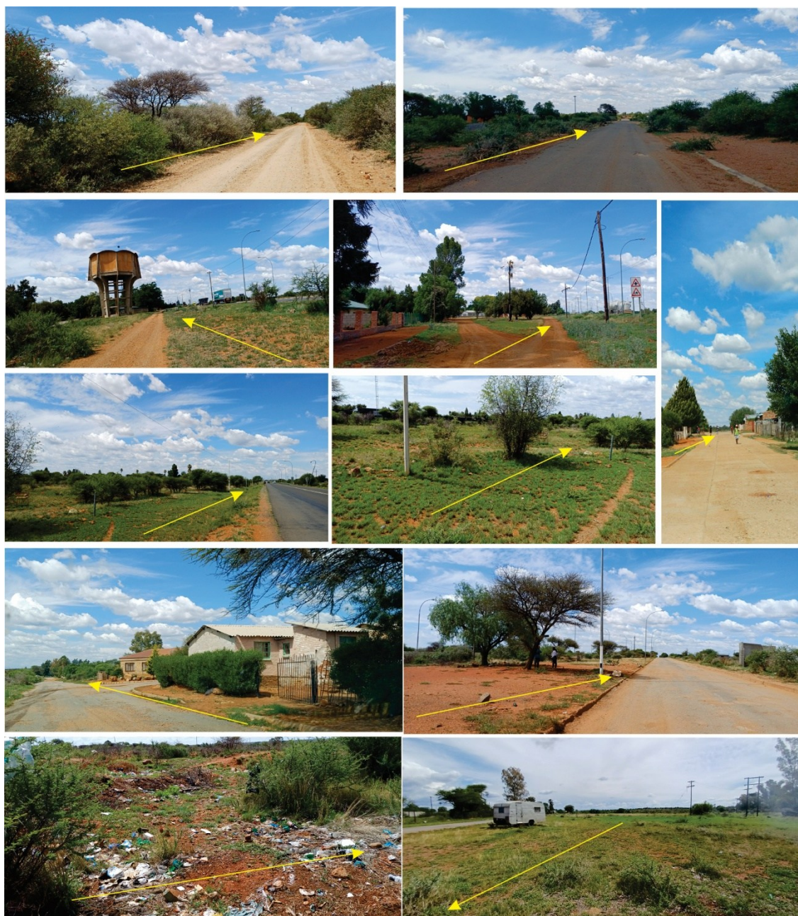
Figure 10. Extensive areas along the Pumping Main, Gravity Line and Rising Main footprints indicate long-term disturbance with much of the route following or intersecting existing tracks, gravel and paved roads, utility servitudes, and cleared corridors, resulting in a high degree of prior modification of the ground surface.
