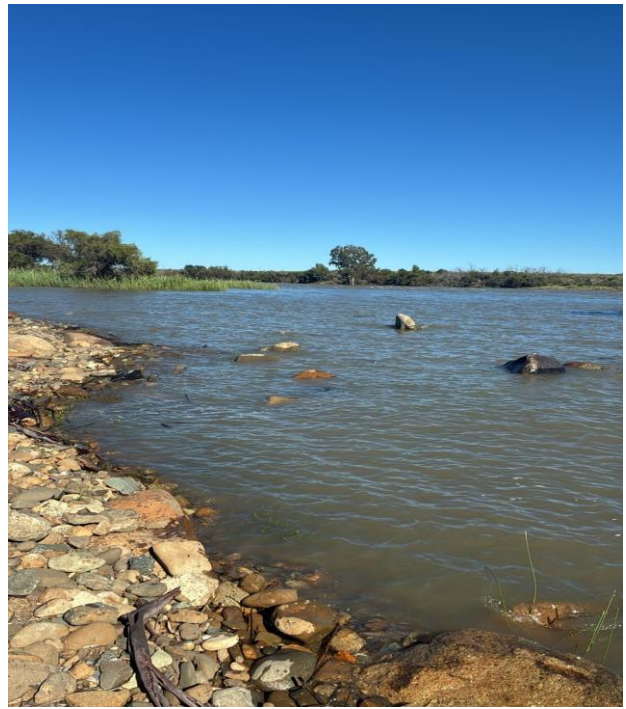
SW01 (Saturation Pond).
